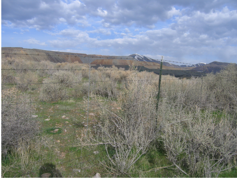
Figure No. 49: Pictured above Midas Creek is the fencing material running along the northern (pictured), eastern, southern and western boundaries of the Lark Tailings reclamation area. The fence is approximately 6 foot with two strings of barbed wired at the top.
