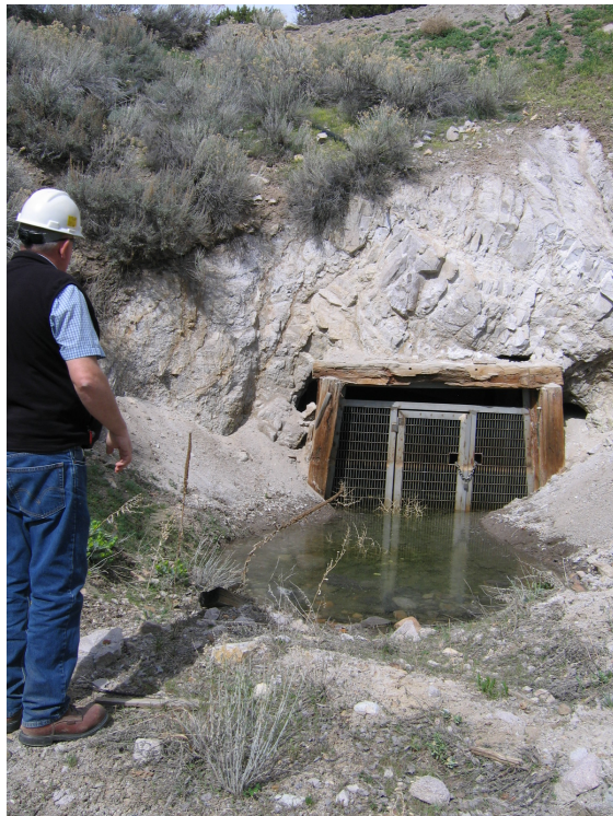
Figure No. 21: Pictured is the Mascotte Tunnel portal, half submerged. The Tunnel is no longer used for ore haulage capacity, but is used to transport water away from the deeper tunnel workings. Mr. Brian Vinton noted that the visible bedrock near the portal is well weathered and crumbly (as can be attested to the fine grand sand left and right of the portal frame).
