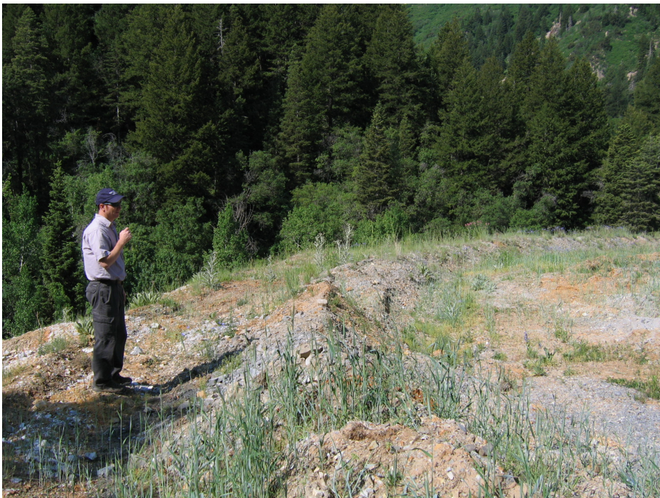
Figure No. 79: Pictured is the water control berm located near the edge of the Water Supply Tunnel Dump's southern embankment (Kelly Payne – Kennecott Project Manager is also pictured). Note the vegetative cover compared to that shown in Figure No. 72 of the August 2005 inspection.
