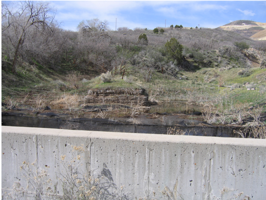
Figure No. 19: Pictured is the Lower Keystone Drainage and cutoff wall. Early response work tried an experimental surface sulfide reducing bioreactor wetland near the wall (black sheeting material) to address surface flows with elevated sulfate; which subsequently was assessed unsuccessful. This cutoff wall is part of the larger Eastside Collection System, which manages potentially mine impacted waters filtering through the up gradient alluvium and flowing surface water. The Eastside Collection System is operated in compliance with a State of Utah Groundwater Pollution Protection permit.
