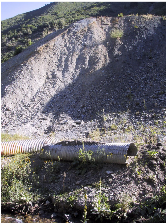
Figure No. 71: Pictured is the Water Supply Tunnel Dump and Middle Canyon Creek from the Tooele County road.
