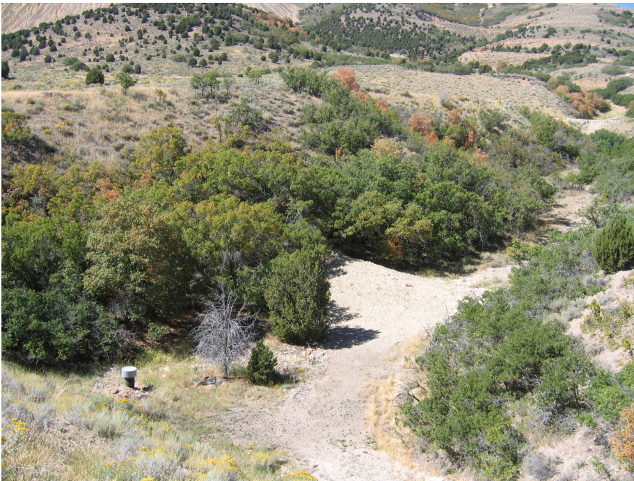
Figure No. 10: Pictured is the upper reach of Yosemite drainage. Note the reconstructed drain near the base of the dam. This area is a desilting basin and the drain allows decant water to flow down Yosemite drainage.
