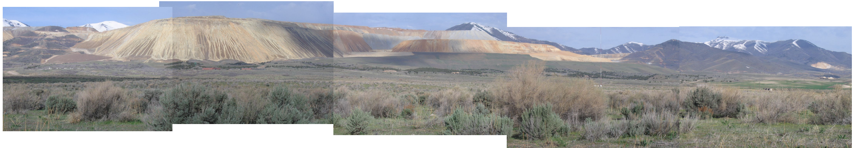
Figure No. 63: Pictured is the top surface of the Lark Tailings reclamation area from near the Southeast Corner. Visible in the distance right side of the panorama is the Midas Creek Silos area (right side of panorama), followed to the left by the white shed and aerial, and followed by the USSRM administration and warehouse buildings in the old town site of Lark. In the far distance are the Bingham Canyon Mine, Eastside Waste Rock Dumps
