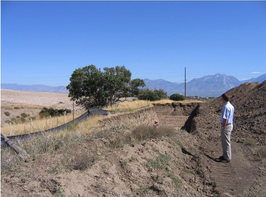
Figure No. 5: Blackhawk development excavation trench or pit.
