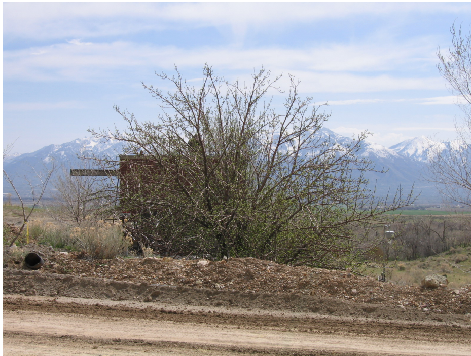
Figure No. 28: Pictured is the Apple Tree sump (behind the apple tree). At the base of the tree is a drop box where Bingham Creek Tunnel and Lark Shaft water combine and are piped to Kennecott's water management facilities near Copperton.
