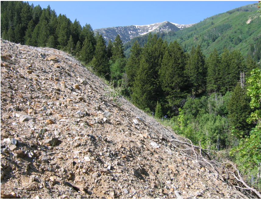
Figure No. 81: Pictured is the western embankment slope of the Water Supply Tunnel Dump taken from the reconstructed drainage channel from the top surface. Some of the slopes along the Dump have seen the successful introduction of voluntary vegetation species, more so than other slopes.
