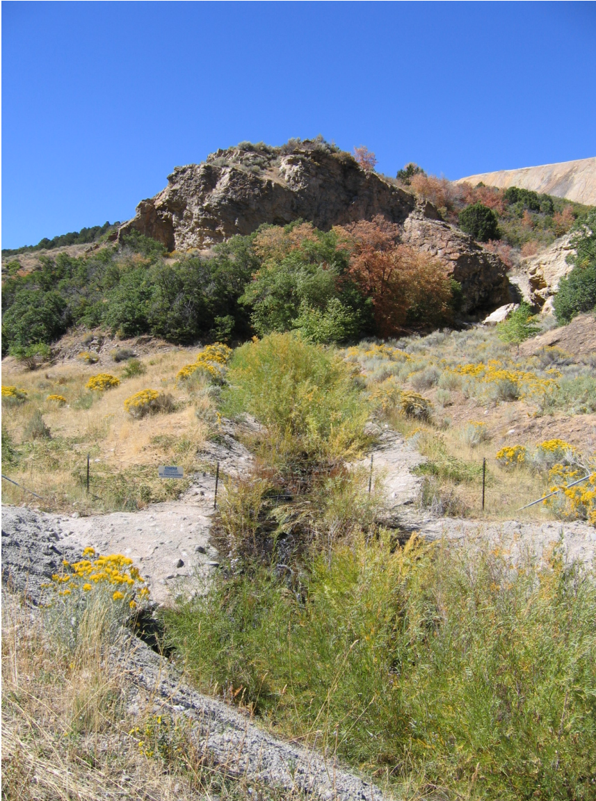
Figure No. 15: Pictured is the adit drain of the Butterfield Mine Tunnel (adit is near rock outcrop). Waste rock was removed from around and near this portal during the removal action.
