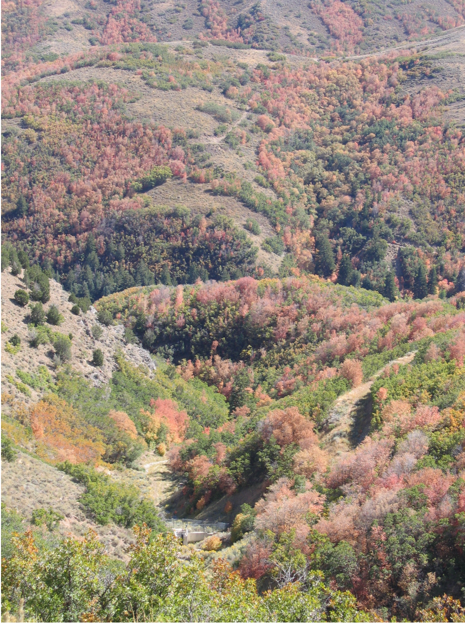
Figure No. 18: Queen drainage just below the Queen Mine site. Pictured is the Eastside Collection System cut-off wall (concrete structure in the first clearing). In the distance and at the base of the drainage is Butterfield Canyon recreational area. Photo was taken from approximately the same vantage point as Figure No. 17.
