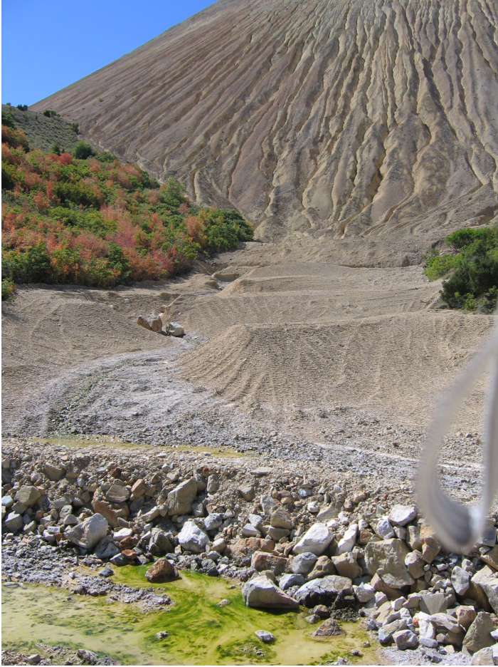
Figure No. 11: Base of Yosemite waste rock dump and reconstructed sedimentation traps.
