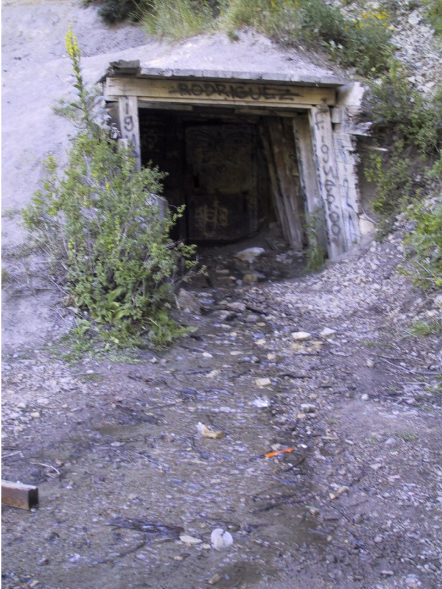
Figure No. 68: In 2005 the Water Supply Tunnel portal remained as historically left by the mine operators. Recessed from the portal front is a steel bulkhead door, which up till 2006 was used to prevent access to the tunnel.
