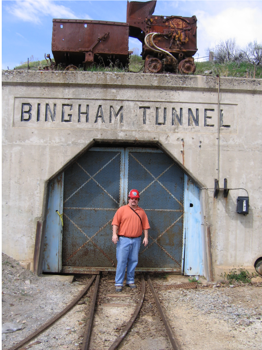
Figure No. 26: Mr. Douglas Bacon (UDEQ project manager) is pictured at the entrance of the Bingham Tunnel. Located in the lower right corner of the photo is a pipe that delivers Lark Shaft water (the Bingham Tunnel intersects the Lark Shaft) to the water management control facilities of Kennecott. The Bingham Tunnel is used today to help dewater the Bingham Canyon Pit; water is taken from the tunnel to another location nearby and then sent via pipe to the water management facilities of Kennecott.
